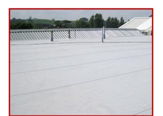
Gables UK Ltd were contracted to install the Kingspan 1000TD, a composite panel system to the newly built hall and kitchen roofs, working with other trades to ensure deadlines were met and work was completed on budget during the school holidays.
