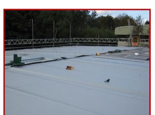
Gables were employed directly by the client to work on a building within a high security area in a sensitive environment. The project involved installation of the Enviroplan single ply waterproofing system, to give a 20 year waterproofing solution.
