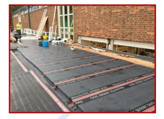
The works to Roof 1 involved the installation of 80mm insulation & a two layer, bituminous membrane, offering a 20 year guarantee.
